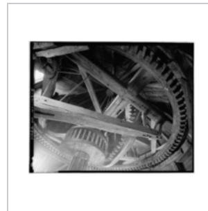
Interior view, Pantigo windmill, East Hampton, New York Historic American Buildings Survey
