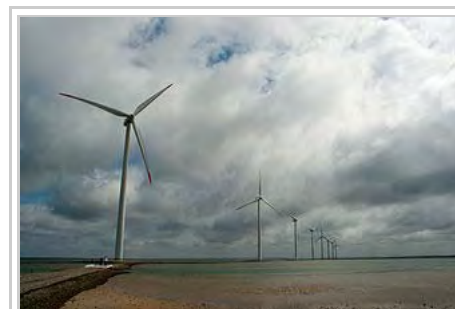
Rønland Windpark in Denmark
