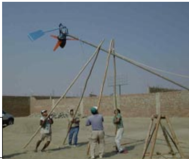
Photo 6 Raising a guyed tower with poles and ropes in Peru (Hugh Piggott)
