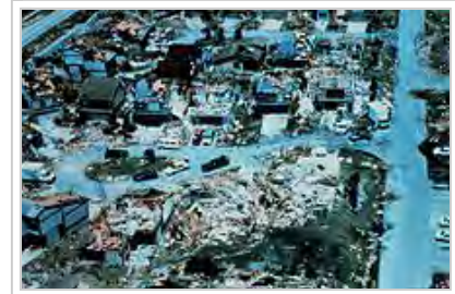
Damage from Hurricane Andrew
