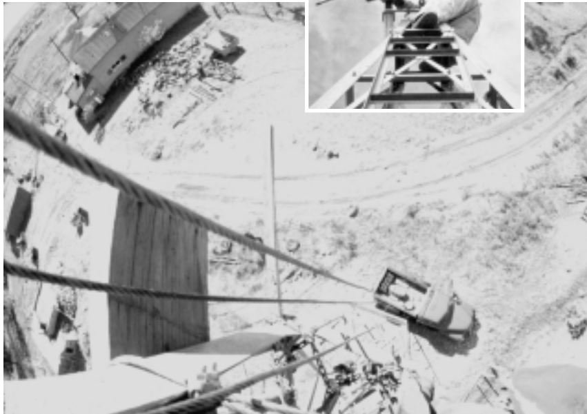
(Right) A Jacobs windplant is wrestled into place atop a tower. (Below) The view from 60 feet up
