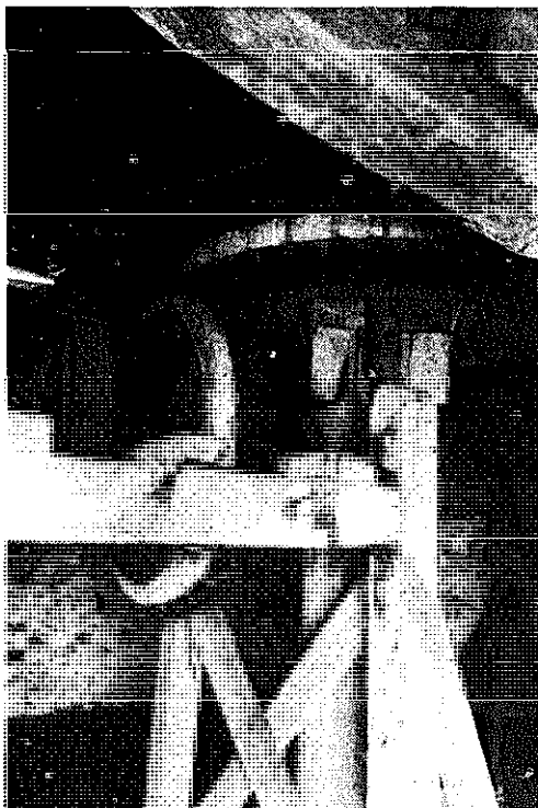
(c) Hickling Tower Mill, Norfolk. Down-turned bevel gear on wooden wallower drives wooden bevel wheel and slack belt
