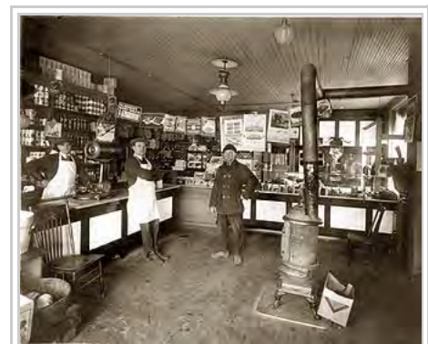
Wood-burning stove heating a grocery store in Detroit (1922)
