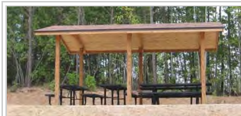
Northeast Park Picnic shelter
