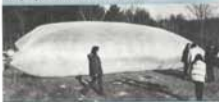
Sheet placed by Carroll team to height 20-ft. 100-ft. sheet of 3-mil polyethylene sheet makes and built dome.
