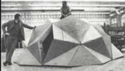
Some in design enough to support tent, and light enough for tent to carry. One gap doesn't seriously weaken structure.
