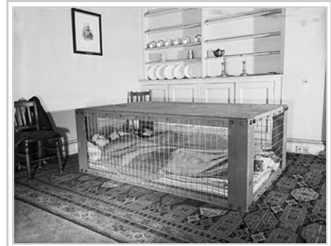
A couple demonstrating the use of a Morrison shelter
