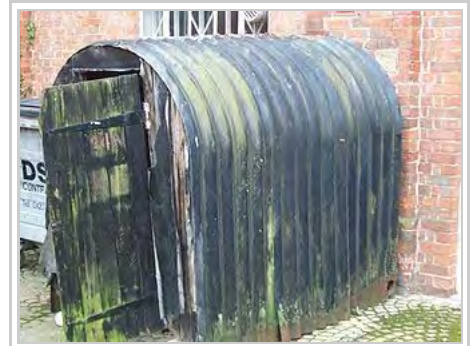
An unburied Anderson Shelter in 2007; this shelter had seen use after the war as a shed
