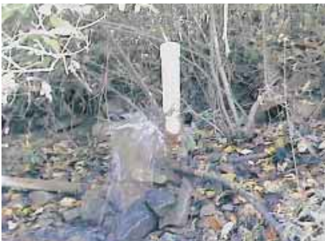
Scott Lee's ram pump in operation.
