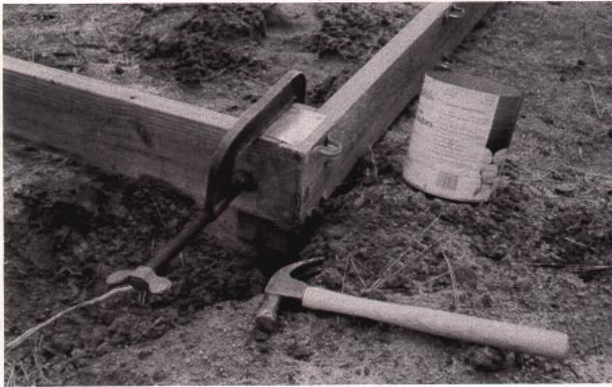
Figure 4. Foundation side and end boards are attached to 4-by-4 posts to anchor the structure. Note the EMT clamps on the side boards hold the PVC pipe ribs.
