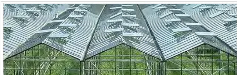
Greenhouses in the Westland region, Netherlands
