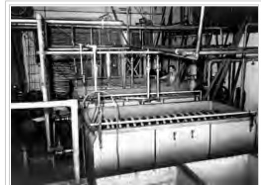
Cream pasteurizing and cooling coils at Murgon Butter Factory, 1939
